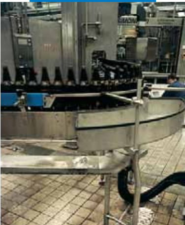
An example of a grouted brewery floor
