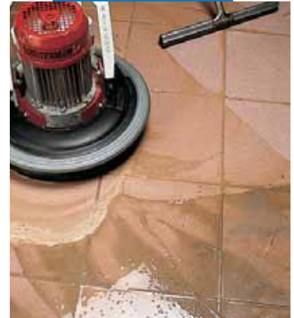
Finishing a porcelain tiled floor with single-brushed power float or rubber squeegee
