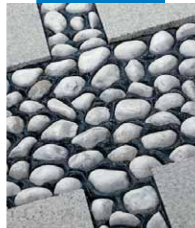
An example of grouted ornamental stones
