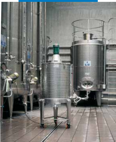
An example of a grouted wine cellar floor
